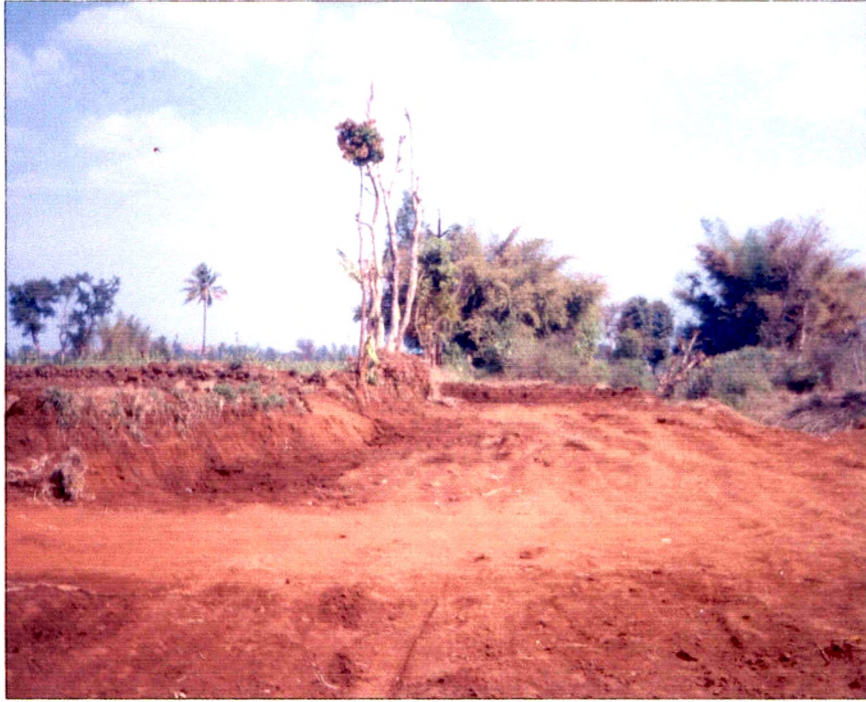
a) Removal of fertile top soil from agricultural field, on river bank at different stages of excavation. (Gandhinagar Site)
