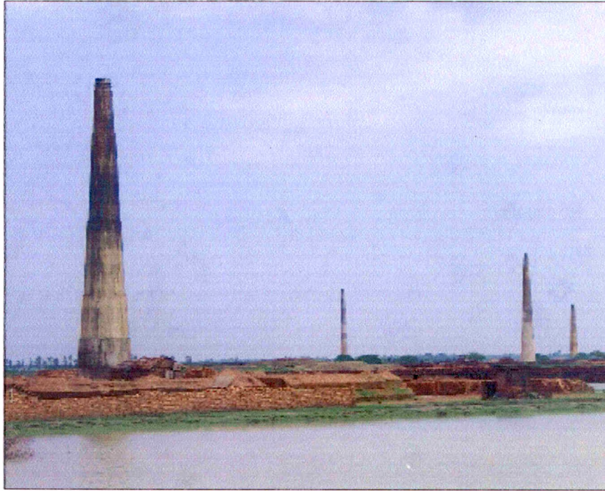
a) Permanent chimney brick kilns in West Bengal. Safer type to reduce air pollution.
