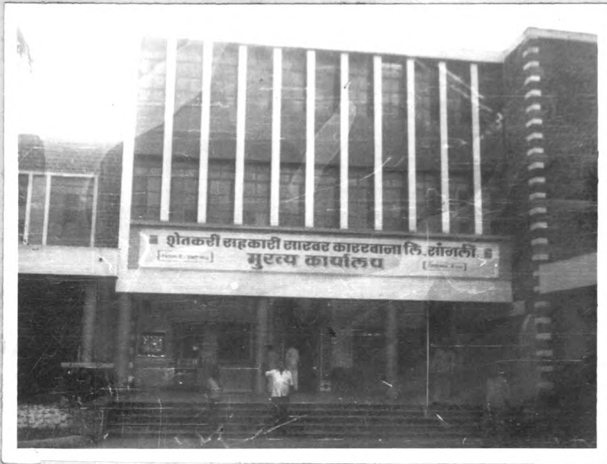
GENERAL OFFICE OF THE FACTORY
