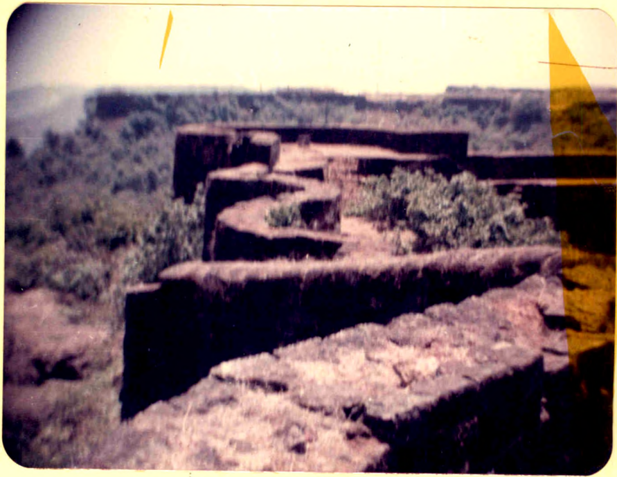
PHOTO.NO.4.B.9 MORTAR WALL
