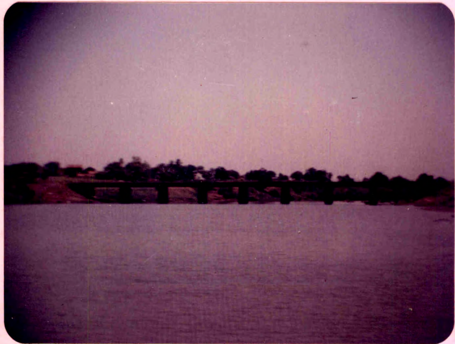
PHOTO. NO. 4. B. 4 KRISHNA BRIDGE
