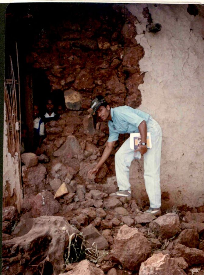
09 Earth quakes...Hit....Hope ? The latest series of quakes raises troubling questions about the stability of the weak houses usually made from mixture of only stone and dried mud.
