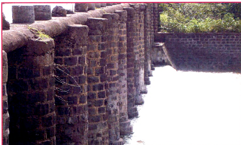
K. T. Weir at Village Arjunwada
