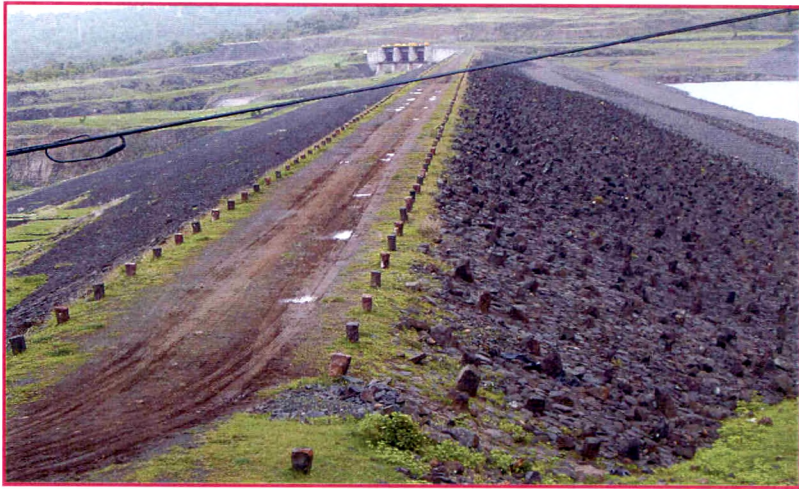
Chikora Dam Site
