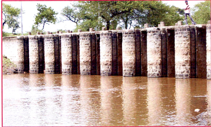
K. T. Weir at Village Galgale
