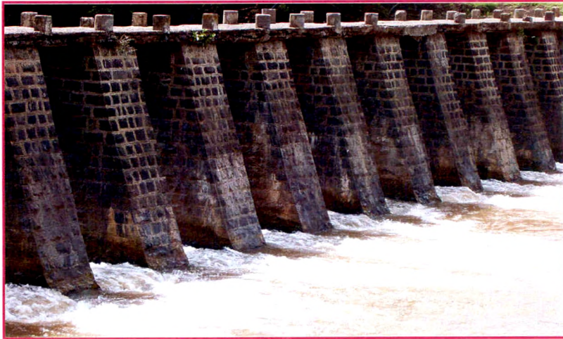
K. T. Weir at Village Metage
