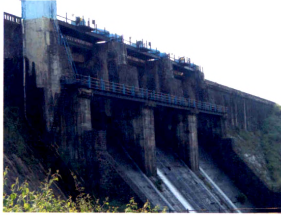
Photo:1 Main wall (48.68 m high &198 m length) and spillway gates of dam.
