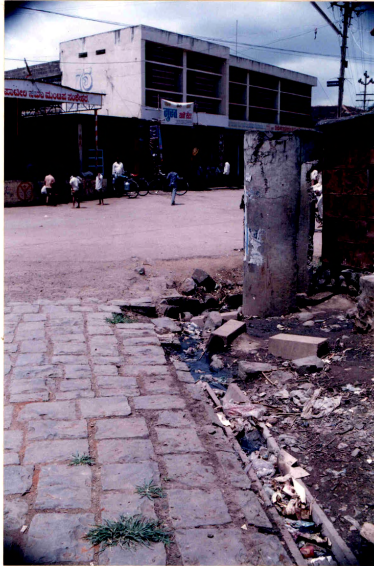
Photograph 4. Dilapidated urinal and the choked gutter with litter (Ward III)
