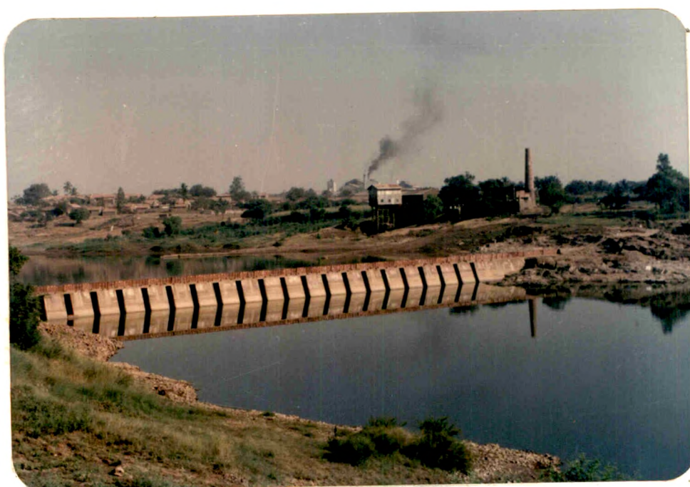
"UGAR DAM ACROSS KRISHNA RIVER AND THE UGAR SUGAR WORKS."
