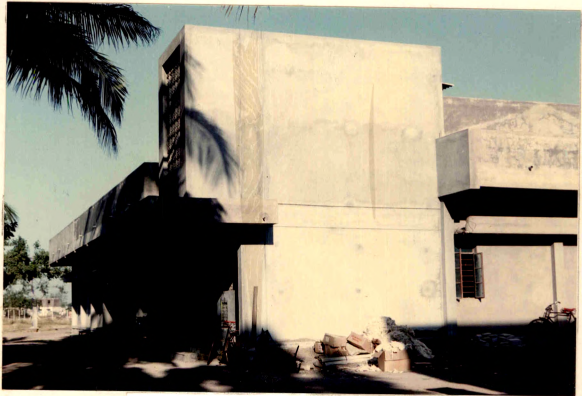
BUILDINGS OF NERLA TUBE FACTORY
