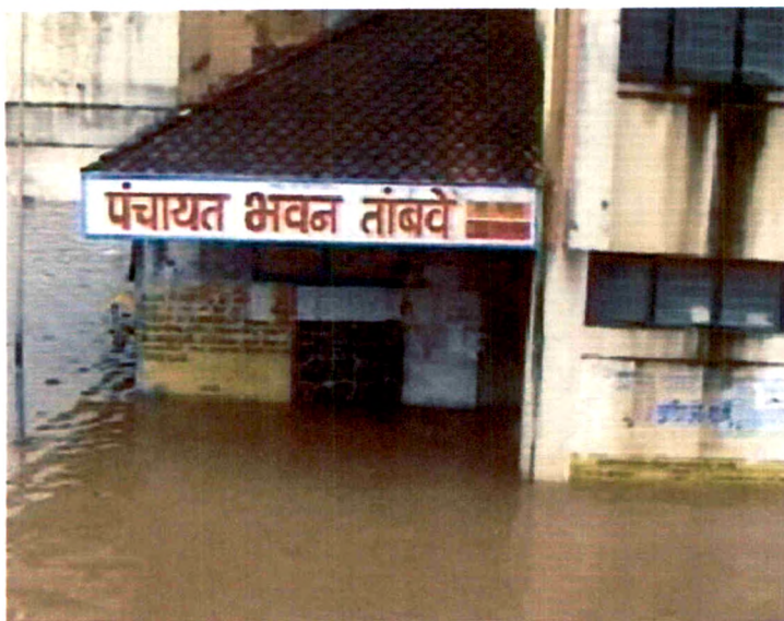
Tambwe Village Panchayat Building half under water
