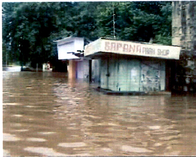
Water Entered into the village settlement
