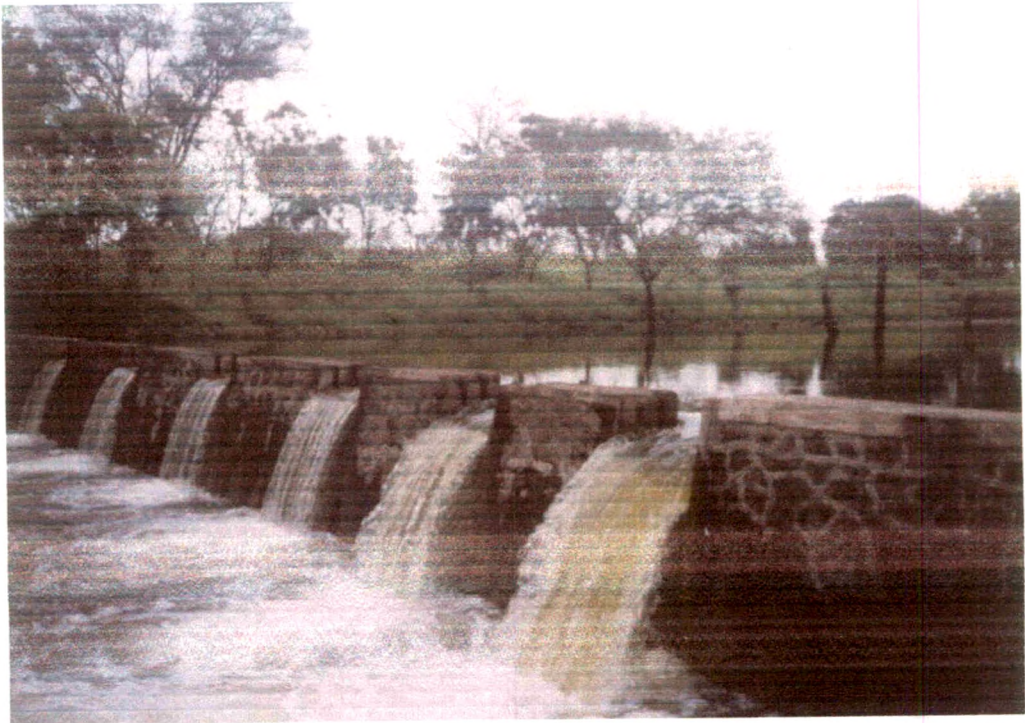
Figure 3.6 Bandhara in the Dhavaleshwar Village
