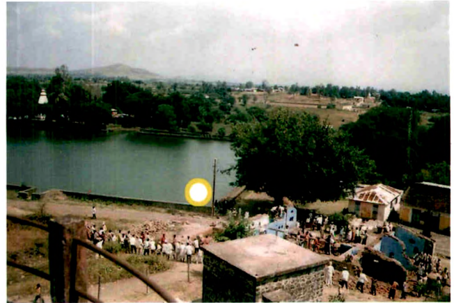
View of 'B' Station of Triputi Reservoir
