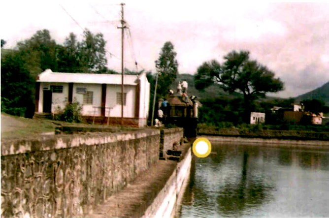
View of 'C' Station of Triputi Reservoir
