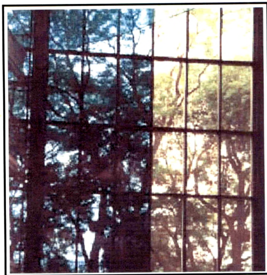
Fig. 1-2. South facing view of a portion of the 8 x 17 m Electrochromic E-Control™ glass made by Flabeg and installed in the Stadtparkasse Dresden am Altmarkt. The left portion of the window is colored. (Source: H. Wittkopf, Flabeg.) [25].
